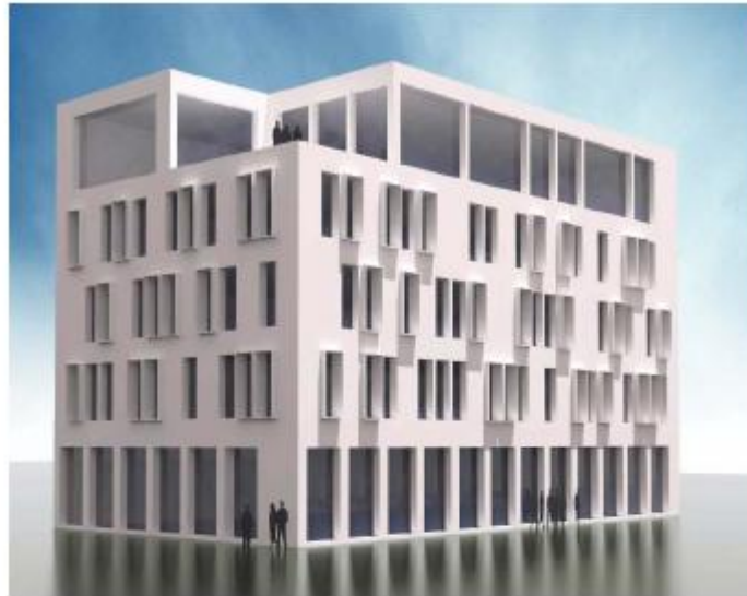
Scenario 1 - BASIC Standard configuration of facade. Reduction of energy consumption of 149,6 kWh/m 2 .
