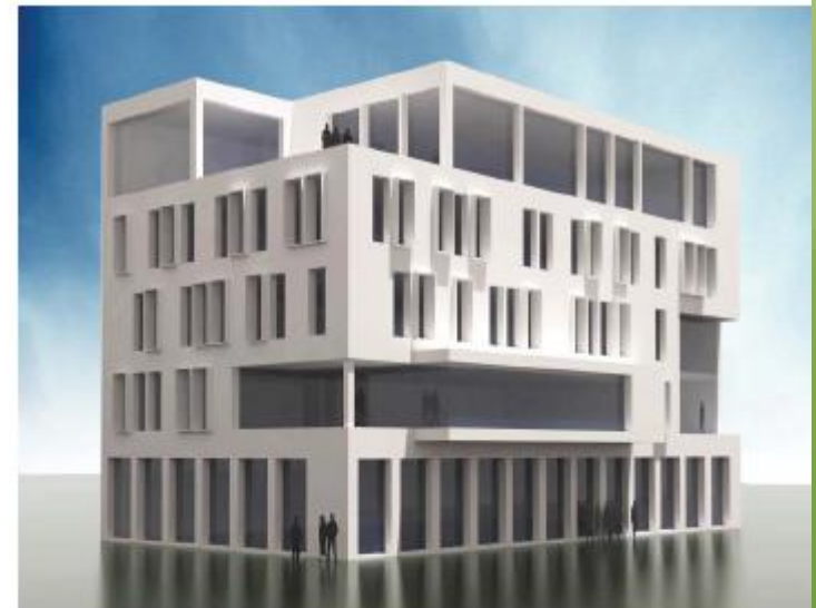
Scenario 2 - FLEX The add-ons and cut-aways are based on the same module as the windows. This allows these elements to be built sustainably and economically whilst also enhancing the aesthetic appearance of the building. Reduction of energy consumption of 67,5 kWh/m 2 .
